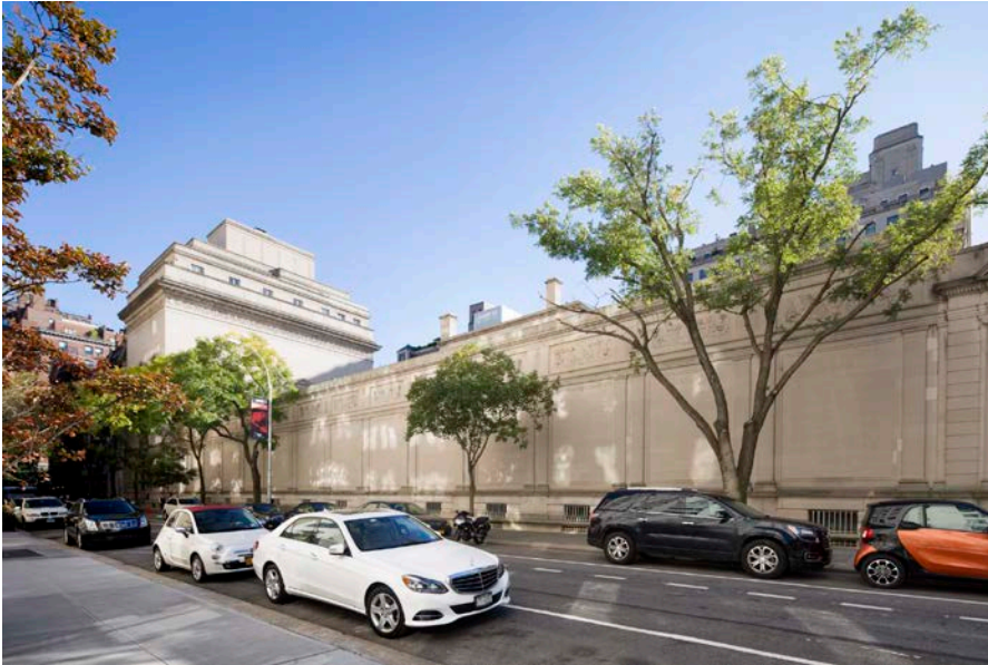
Current view of The Frick Collection (with Frick Art Reference Library building to left) from Fifth Avenue and 71st Street; Courtesy of Selldorf Architects*
